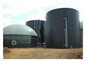
Figure 3 Commercial anaerobic digester using cow manure and industrial waste, Source:
